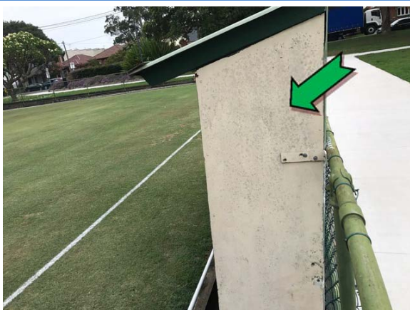
Photo 5. Exterior north west elevation hut, wall – non asbestos-containing fibre cement sheeting.
