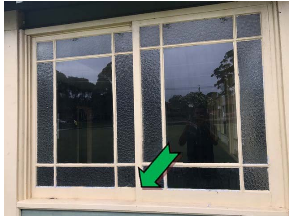
Photo 4. Exterior, throughout, window frames – non asbestos-containing window caulking.
