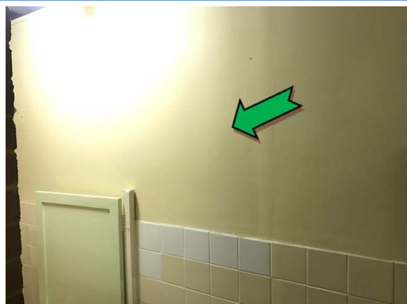
Photo 6. Interior, ground level, male toilets, wall – non asbestos-containing fibre cement sheeting.
