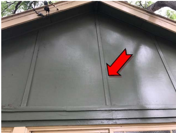
Photo 3. Exterior, western elevation, gable end – assumed asbestos-containing fibre cement sheeting.
